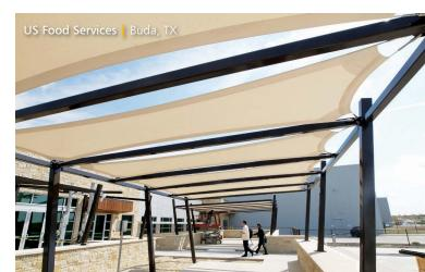
Tension structures or tensile structures, are architecturally innovative forms of construction art that provides designers and end users a variety of aesthetic freeform canopy designs utilizing membranes such as PTFE-coated fiberglass or PVC. Tensile fabric structures offer a variety of functional benefits including exceptional daylighting and durability, flexible design capabilities, lightweight nature, minimal maintenance, cost efficiencies, and a range of membrane choices.
